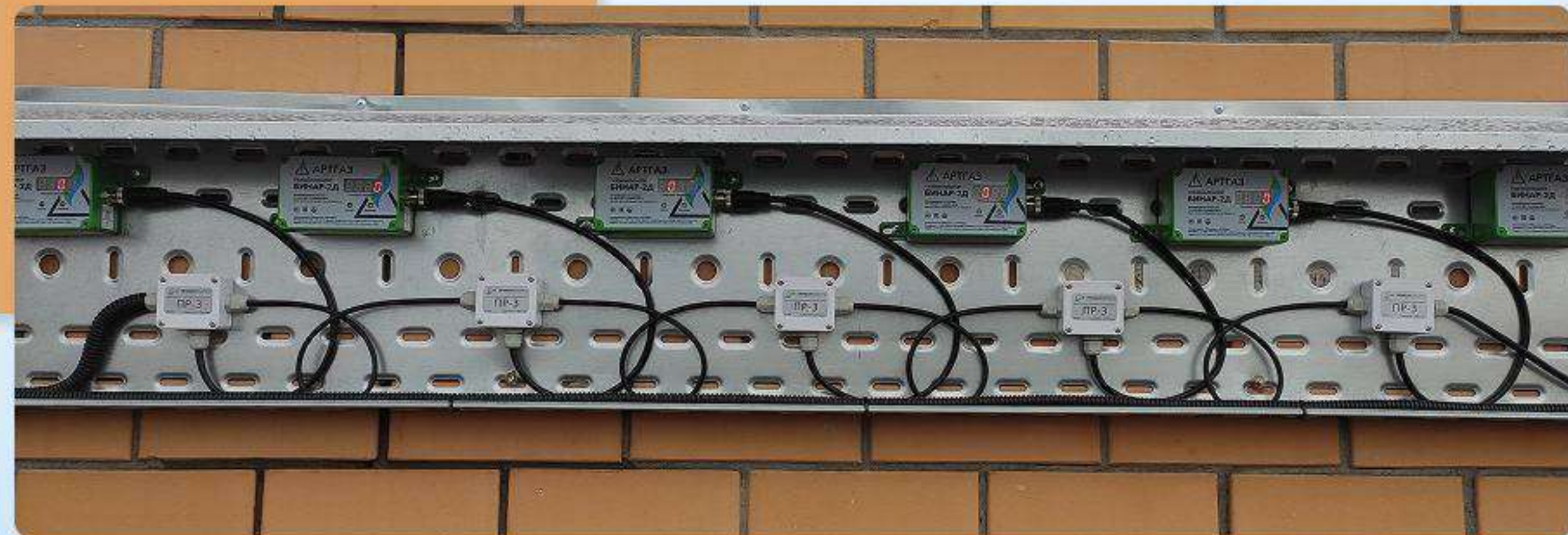
Installation of a weather station, sensors and gas analyzers
